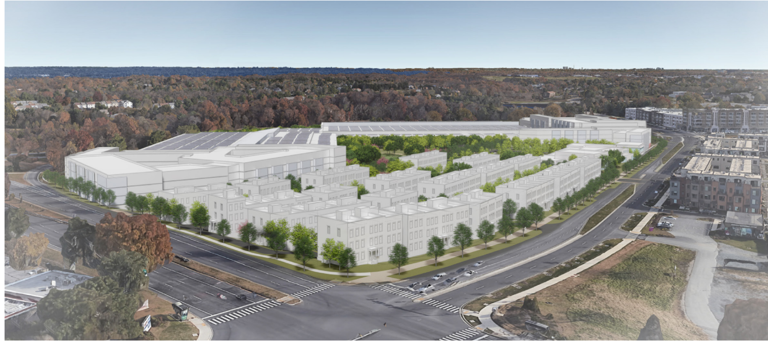
VIEW LOOKING EAST, FROM SHADY GROVE ROAD
