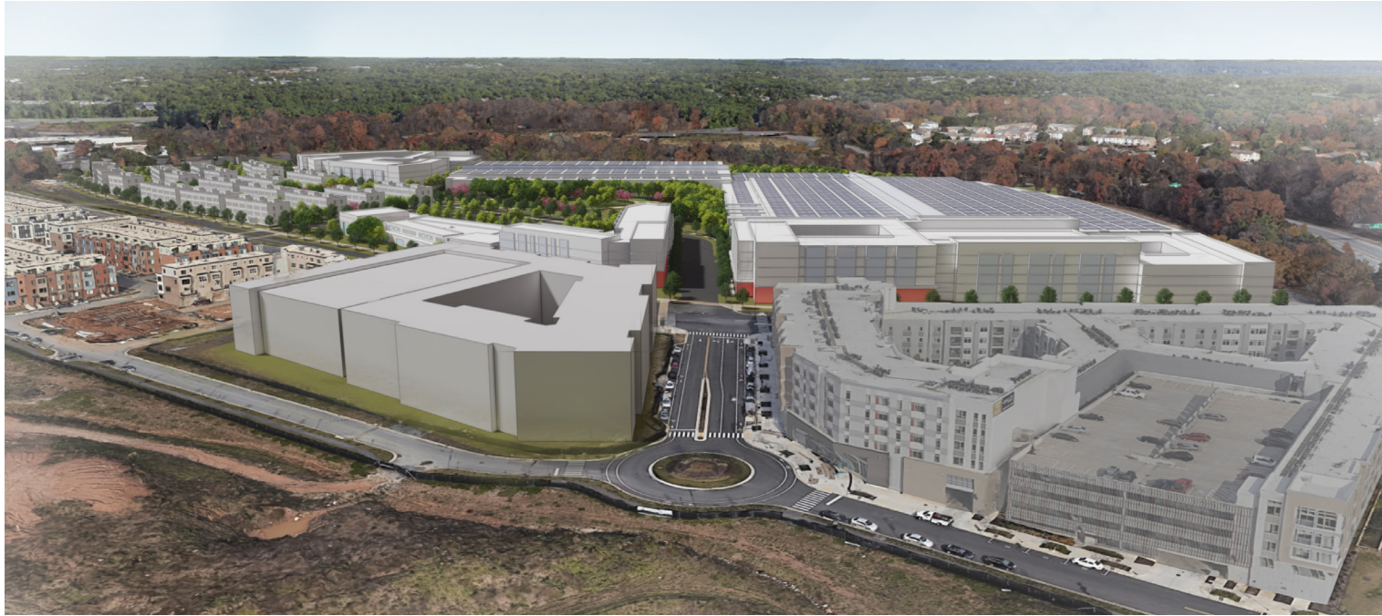
VIEW LOOKING NORTHEAST, OVER WESTSIDE MULTI-FAMILY AND GRAMERCY BLVD.
